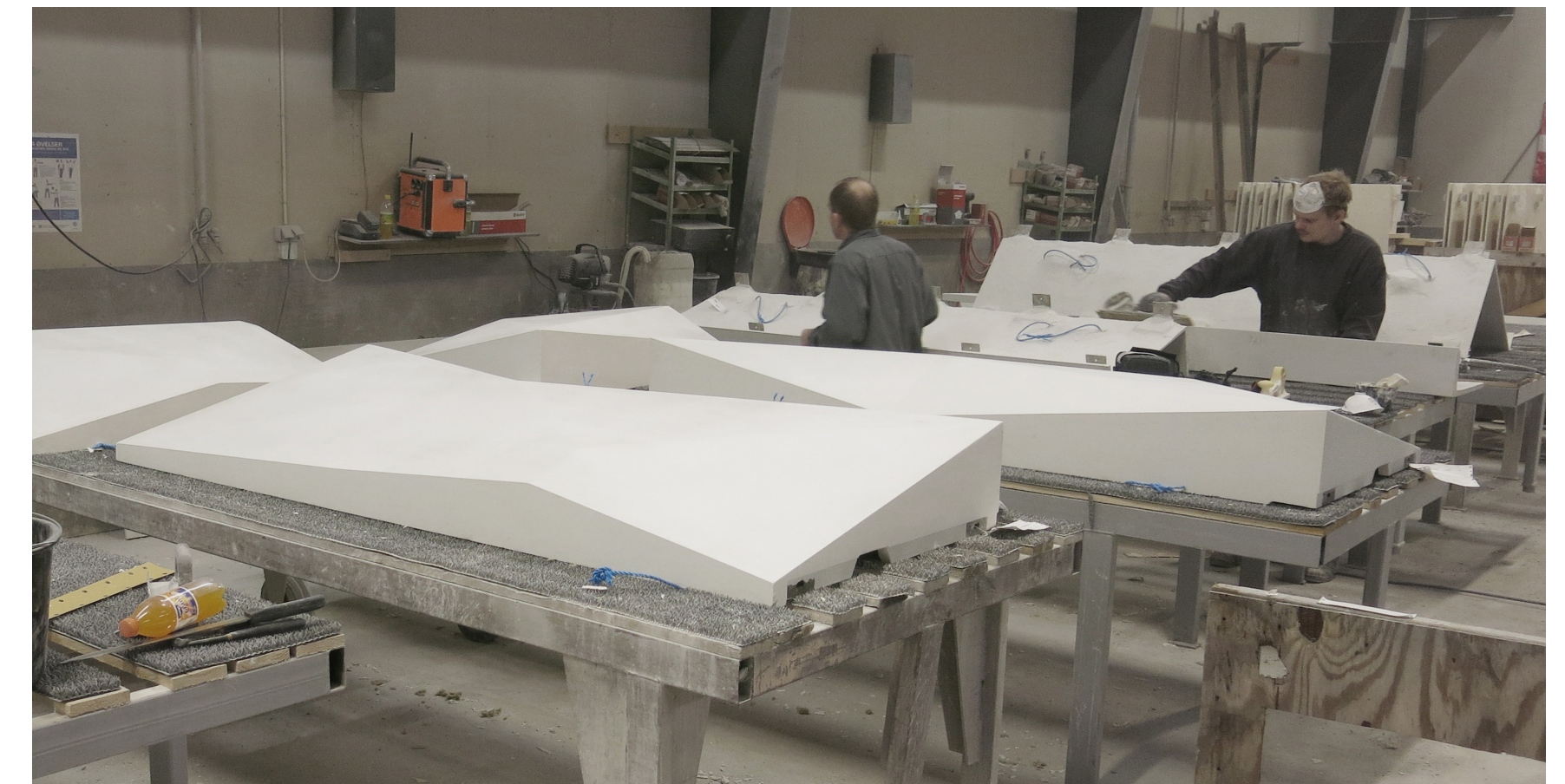
concrete spraying and element demoulding
