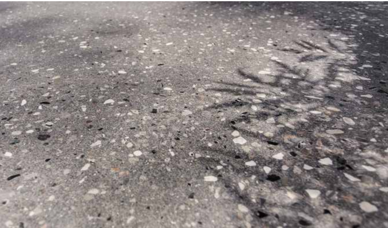
Genbrugsbetongulv i CPH Towers' foyer
